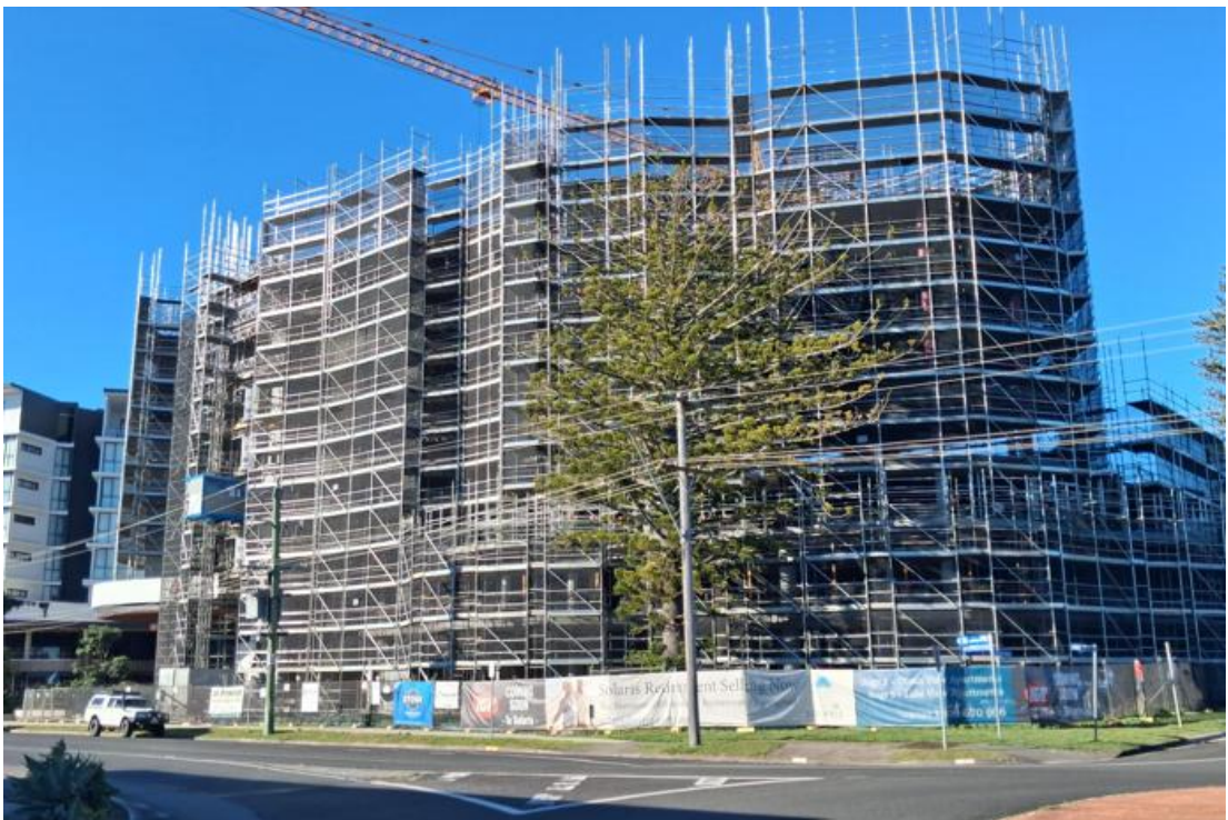
Plate 2 –Existing Site Conditions - Stage 2 (Building B) under construction (Northern Elevation)
