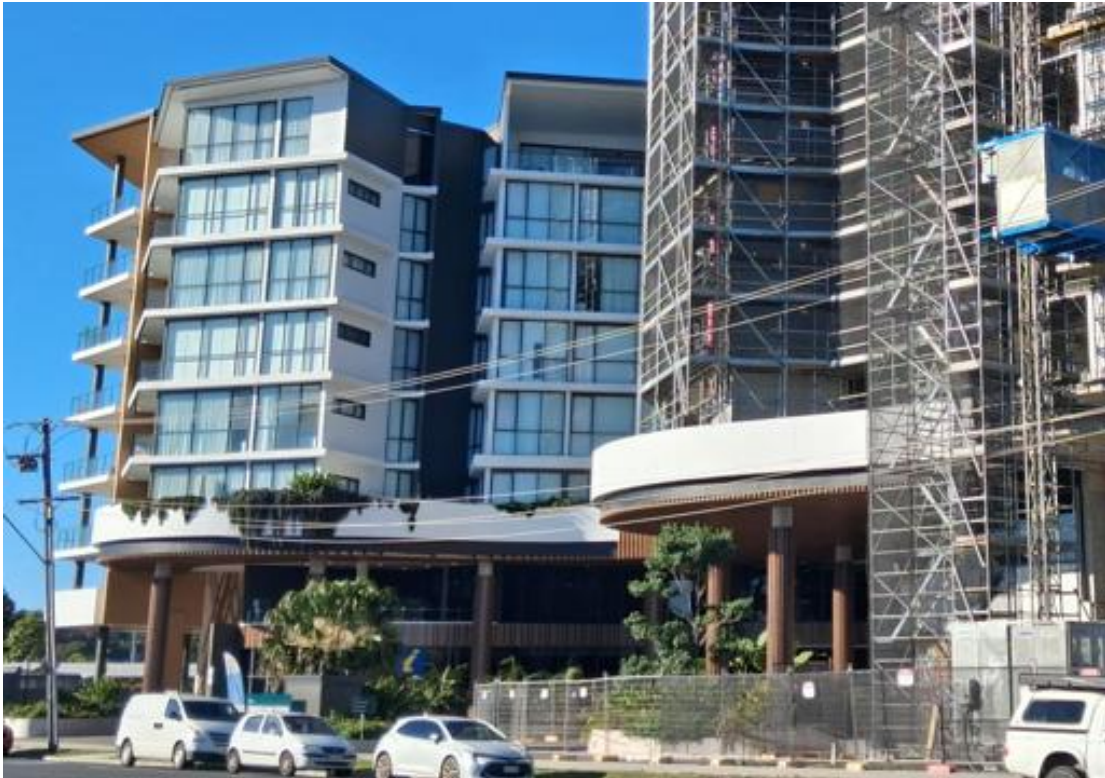
Plate 1 –Stage 1a, 1b & 1c (Building A) completed (Northern Elevation)
