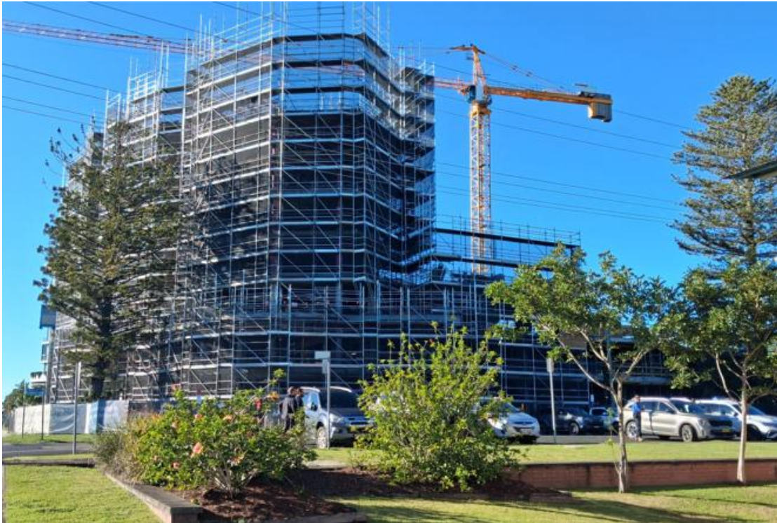
Plate 3 –Existing Site Conditions - Stage 2 (Building B) under construction (Western Elevation)
